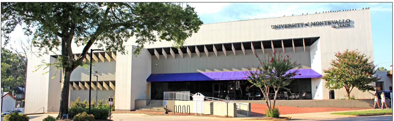
Arguably the most dramatic example of modern architecture in Montevallo is the 1977 Alabama Power building on Main Street. Today it is the University of Montevallo on Main. It was conceived to test the viability of solar power, thus it's orientation to the sun.
