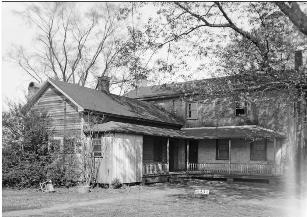
(Left) A mantelpiece in King House documented by the HABS photography in 1934. (Above) This HABS photo shows a rear view of the King House and how at some point in its life the original detached kitchen building had been taken down and replaced by attached kitchen and porch additions.
