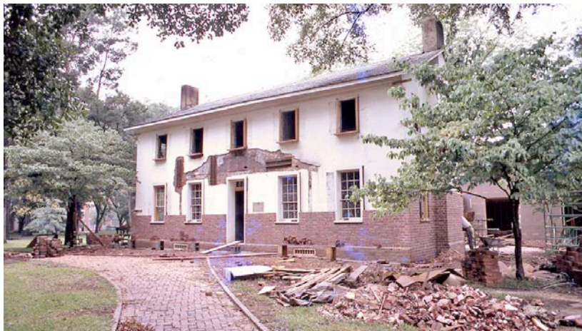
A layer of new brick was laid over the old stucco and original brick veneer.
