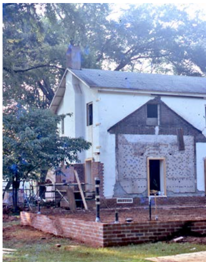
The original profile of the house emerges after removal of the addition.
