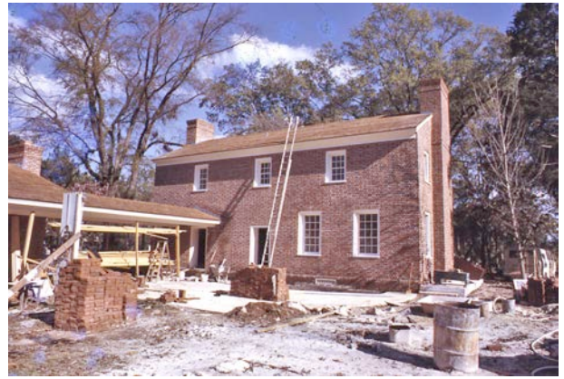
The original detached kitchen was recreated and connected to the house by a covered walkway.
