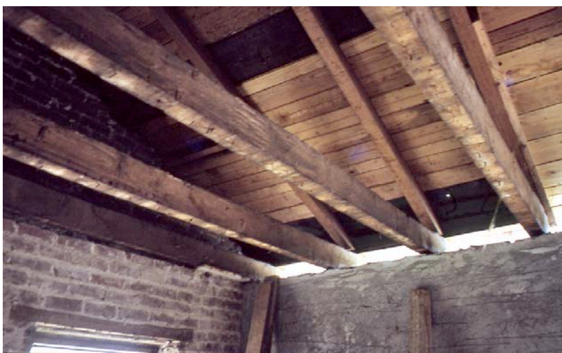
Rough hewn 1820s-era rafters were also discovered as the house was carefully taken apart during the initial stages of the restoration process.
