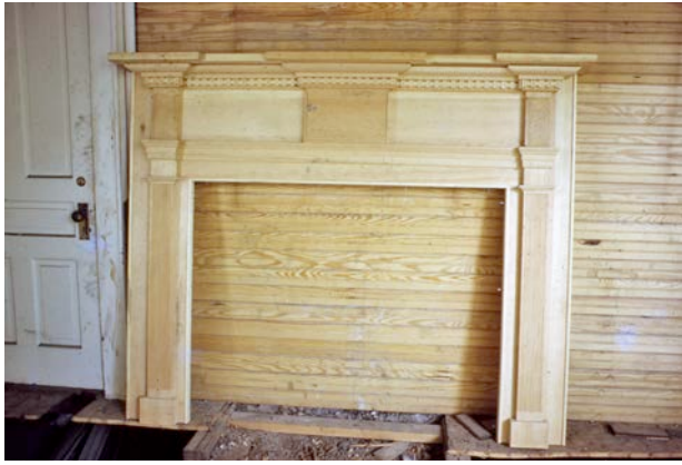
This mantelpiece was original to the house. It was sent away to be stripped and returned for reinstallation.
