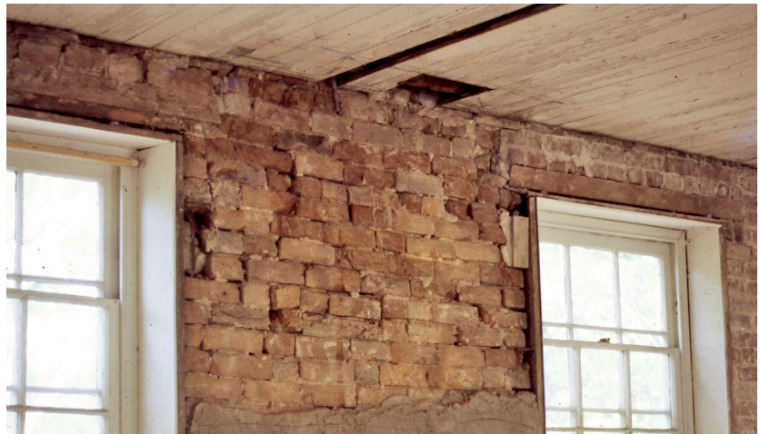
A revealing example of the homemade bricks used in the construction of King House along with the crude patterns and materials employed in laying them.
