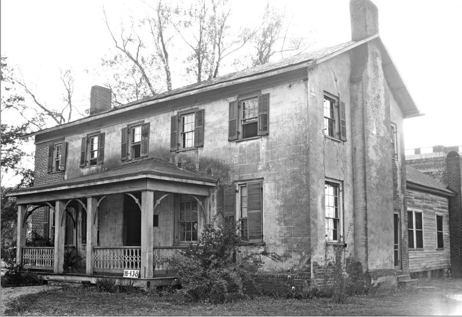
The Historic American Buildings Survey (HABS) sent a photographer to Montevallo to evaluate and make photographs of the 111 year old building as it looked in 1934. The photo clearly shows how the stucco, applied following construction to protect the original brick from deterioration, was scored to create the illusion that the house had a veneer of large blocks of stone.
