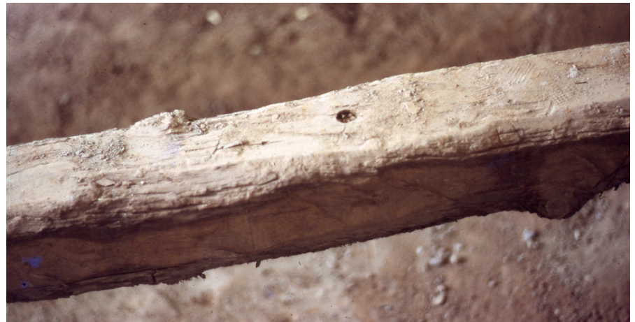
The rudimentary woodworking tools used to shape and prepare this timber for use can be discerned from the variety of markings they left in the wood.
