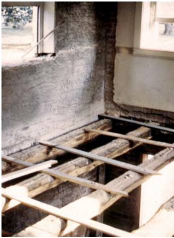
Floor joists exposed and ready to support the new floor.
